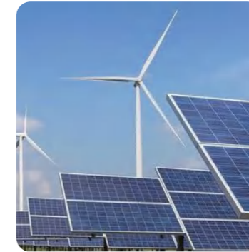
Wind-solar hybrid power generation
